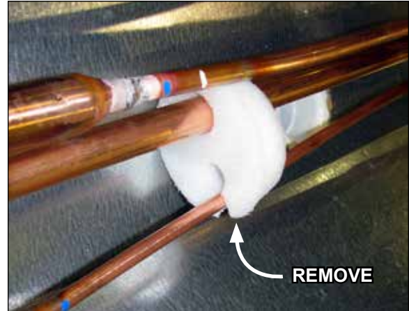
Fig. 6 Remove the shipping blocks
